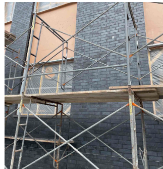
Exterior brick placed outside of the building.
