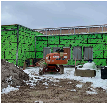
Exterior sheathing on the building.
