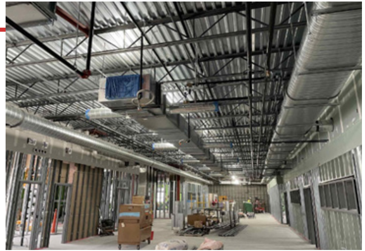
Mechanical duct work being completed in the classroom wing.
